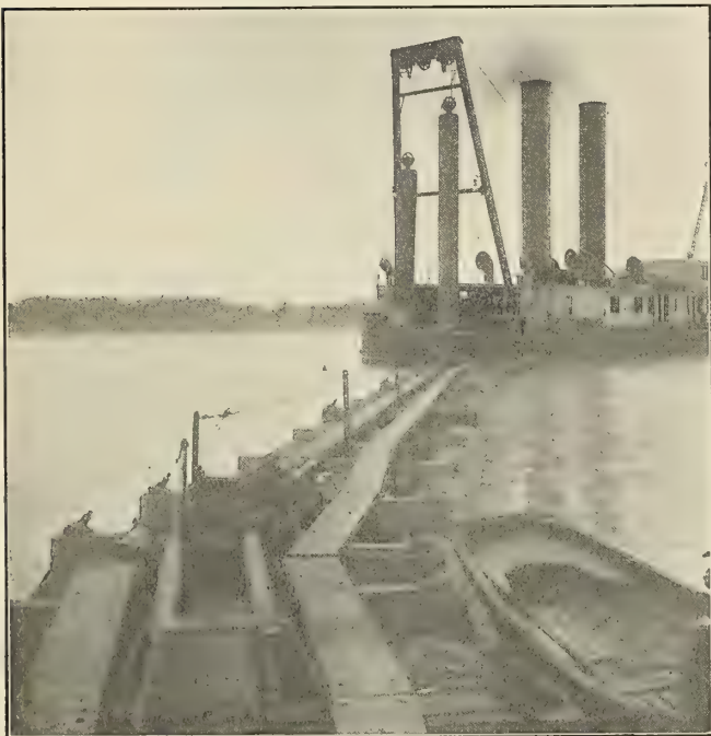
THE PONTOONS AND PIPE-LINE SUPPORTS.
